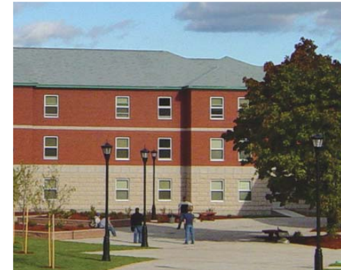
Only 1150 man hours were required to install 14,393 sq. ft. of ICF wall area enclosing this 30,400 sq. ft. building.
